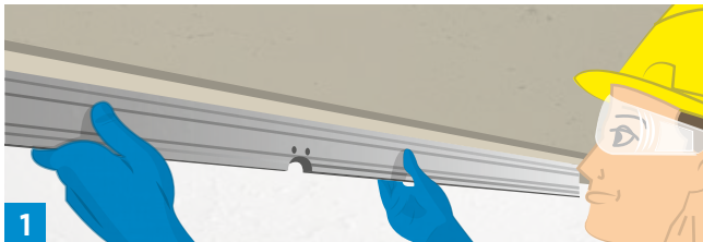
1 Verify that the supporting construction is level.
